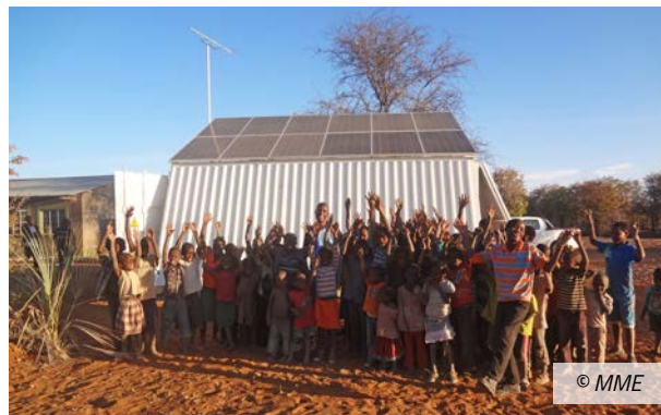
Containerized PV System improving access to energy for government institutions and households in Namibian rural areas.
